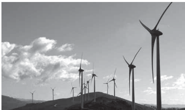
Figure 15 Europe's biggest onshore wind park in the northern region of Viana do Castelo, Portugal. Photograph: Estela Silva/EPA.
