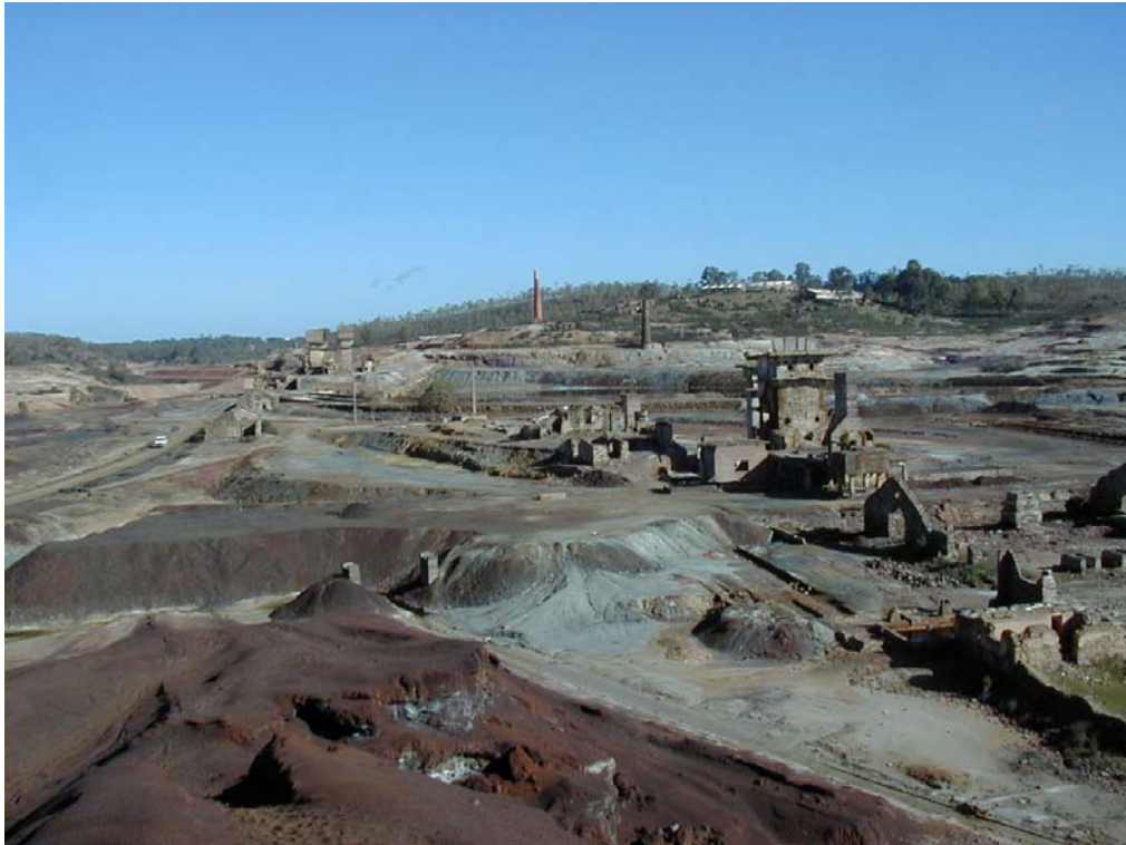
Figure 6. Achada do Gamo: remnants of mining infrastructures and dispersed or concentrated waste mining material.
