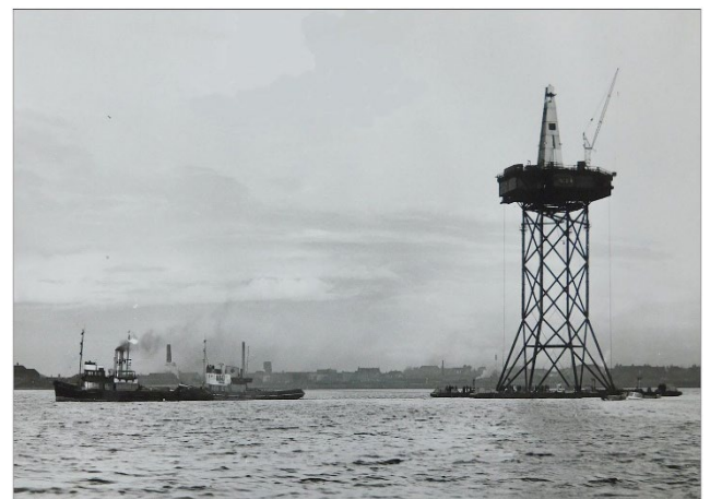
Figure 2. The National Coal Board's Second Off-shore Drilling Platform (Tower) being towed from the Port of Hartlepool to its boring position off the Durham coast ( National Archives, Kew, London. Coal 80/1096-42 ).
