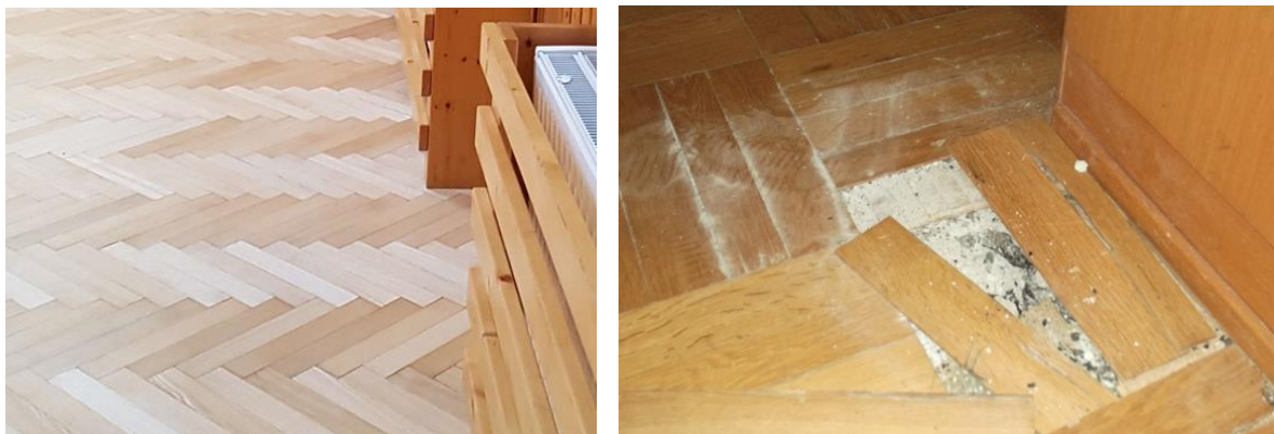
Figure 7.15 - Checking quality and reuse potential of parquet floor in building to be demolished (BauKarussell, 2018).
