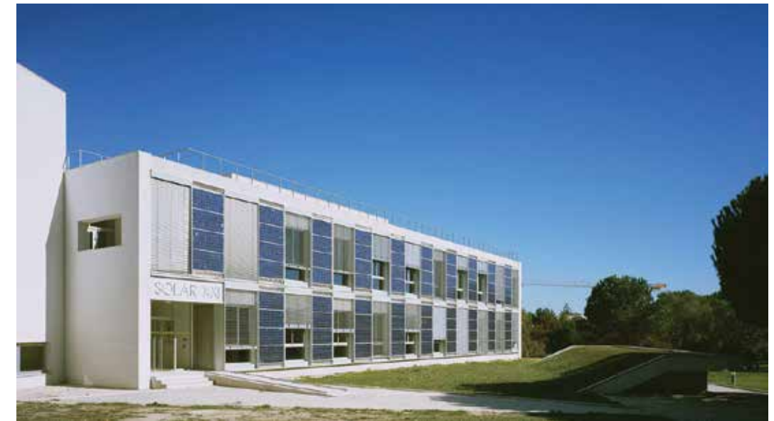
Fig. 8 Solar Building XXI in Lisbon (Portugal).
