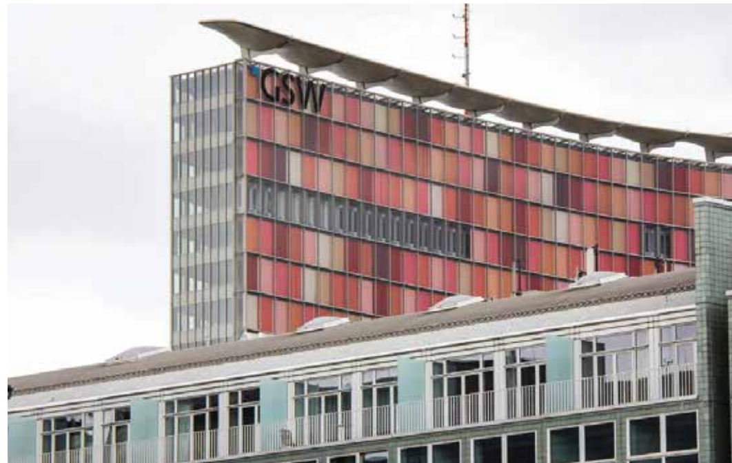
Fig. 7 Façade example, GSW Headquarters (Sauerbruch Hutton) in Berlin (Germany).
