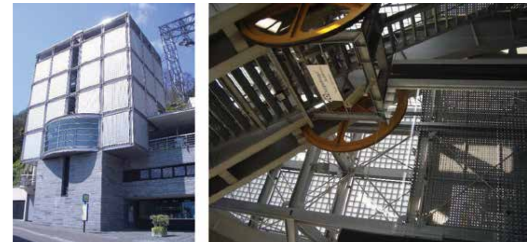
Fig. 2 Station of the Orselina-Cardada cableway, Locarno, a) Front view, b) Internal steel structure of the station.
