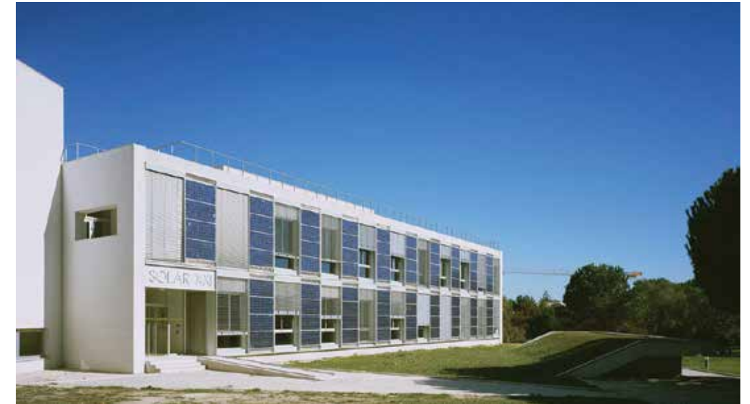
Fig. 8 Solar Building XXI in Lisbon (Portugal).
