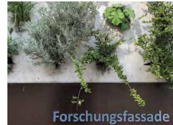
Fig. 9 Detail of the Green Façade at the Frankfurt University of Applied Sciences
