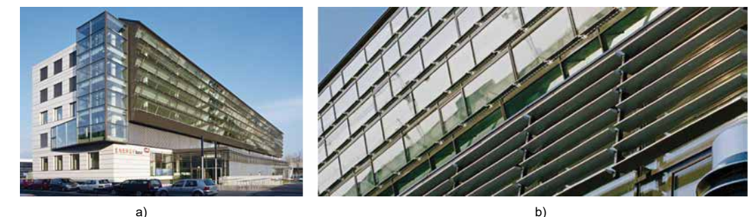
Fig. 6 a) ENERGYbase building (Architekten ZT KG, Vienna, Austria). b) Detail of the South façade.
