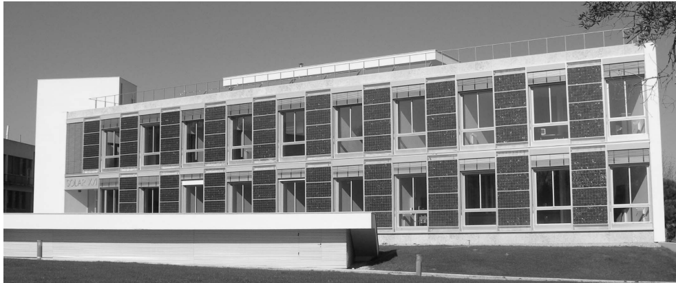
Figure 1: Direct gain and PV panels in south façade of Solar XXI building. Architects: Pedro Cabrito and Isabel Diniz.
