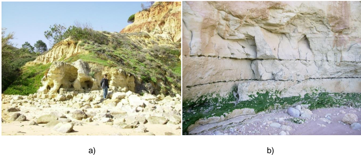
Fig. 2.4 – a) Top: reddish Plio-Quaternary formations; Middle: yellow detrital fine carbonate sandstone from Miocene; Bottom: yellow carbonate Miocene with intersected pipelines. b) Dissolution on bedding planes and joints of the Miocene.
