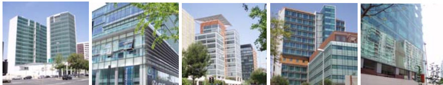
Fig. 1. Service Buildings (Lisbon).
