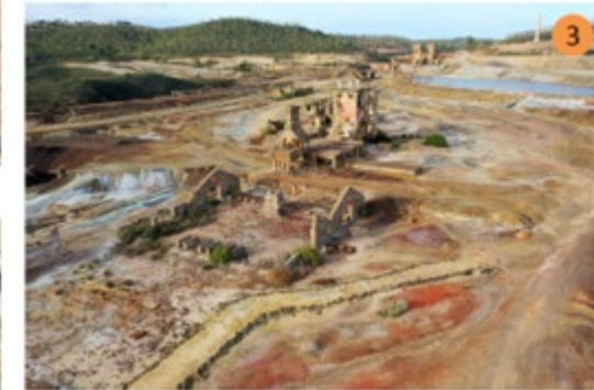
Achada do Gamo | Sulphur factory
