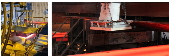
Figure 20 - RGS Thermagy integrated in (Left) glass industry and (Right) in a typical steel plant.
