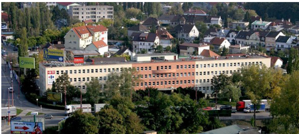
Figure 27 - Headquarters of the State Geological Institute of Dionýz Štúr in Mlynská dolina in Bratislava.
