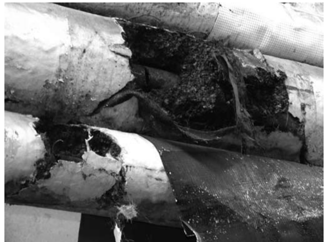
Fig. 4. Cooling pipes with ICB insulation before demolition.
