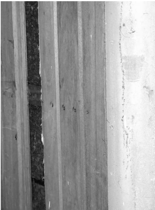
Fig. 3. Detail of ICB behind the wood paneling protection (wall insulation).
