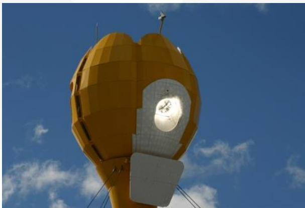
Temperature in the Tulip micro turbine is 1000 degrees Fahrenheit
