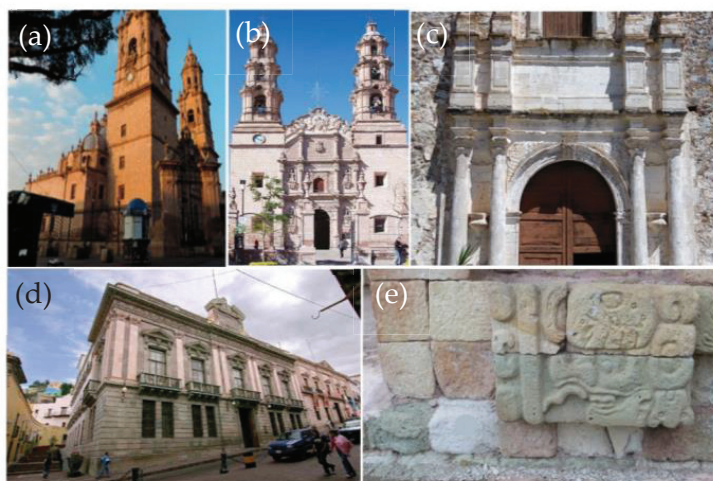
Figure 4. Examples of representative tuff-built AHSs in North America: (a) Cathedral of Morelia, Mexico, (17th century) [42]; (b) Cathedral of Aguascalientes, Mexico (16–20th century) [16]; (c) Façade of Santa Veracruz Chapel of Mineral del Monte, Mexico (16th century) [46]; (d) Façade of Legislative office, Loseros, Mexico, 19th century [45]; and (e) Maya tuff stones, in Archeological Site in Copan, Honduras, (763 CE) [47].
