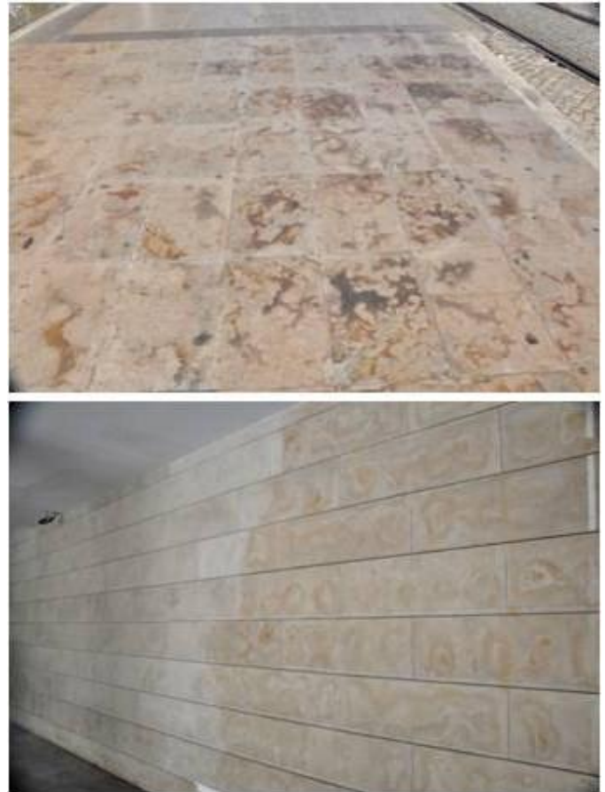
Figure 1 — Example of stains in limestones applied in pavements (up) and cladding (down).
