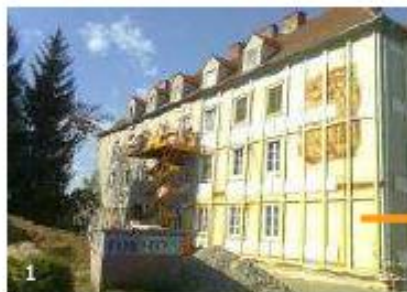
South oriented facade of the long building row
