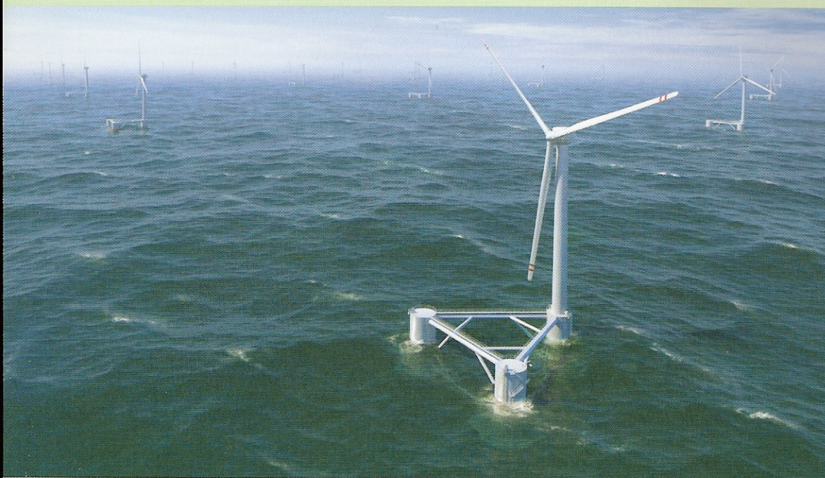
Figure 5 The WindFloat structure
